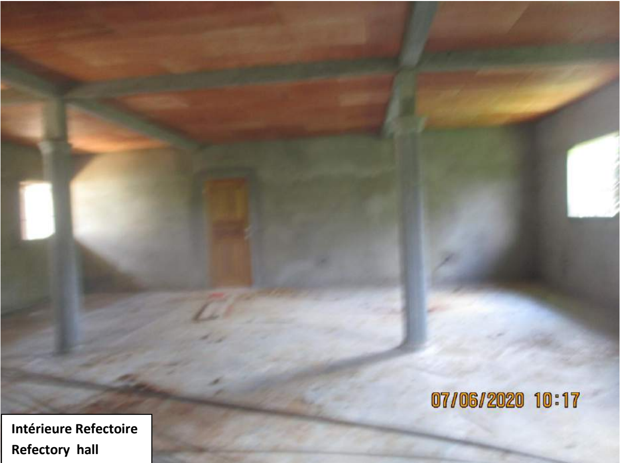
Batiment Refectoire et cuisine Refectory hall and kitchen
